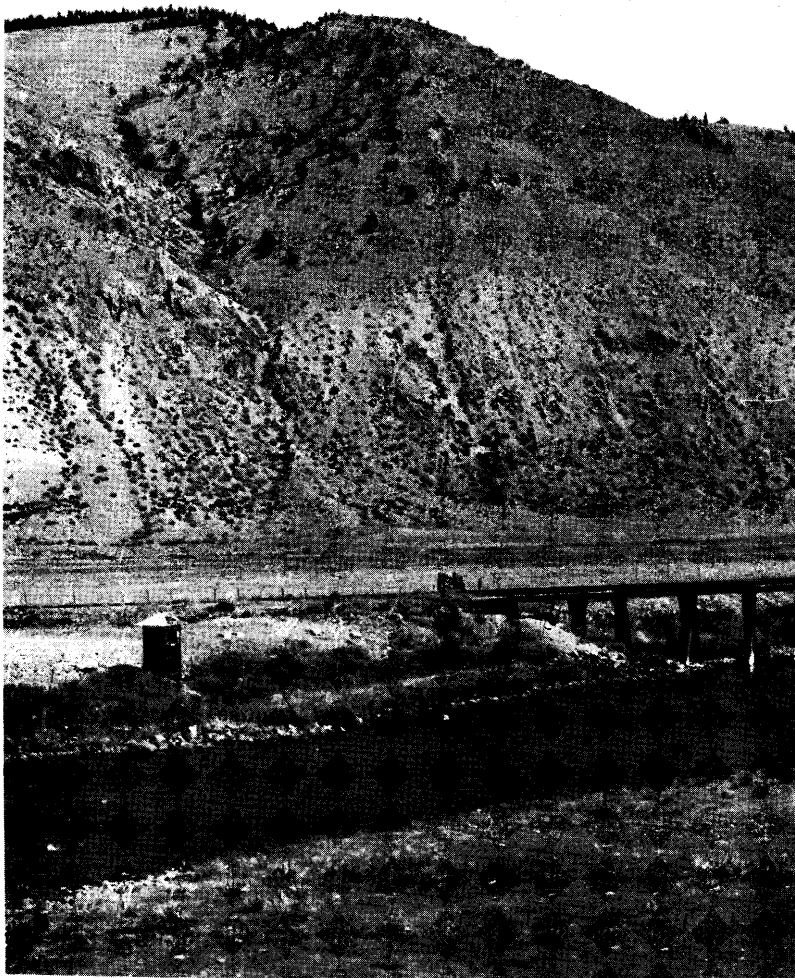
Figure 2.3 A patriarch of the gaging network: Rio Grande at Wason, below Creede, Colorado. The station was established in 1907 as a staff gage. The house seen here was built in 1910. A recorder was installed, and a cable was built at the gage house. When the station was discontinued in 1954, Lisle Alsdough of Del Norte moved the cable to another location.
